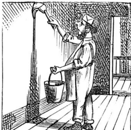
Common lodging-houses to be white-washed this week.
